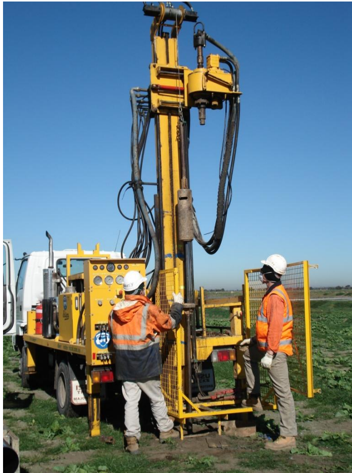
Figure 1 : Standard Penetration Tests (SPT) carried out on site
